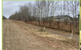
Electric fence and steel fence encroachment into trail clearance zone
