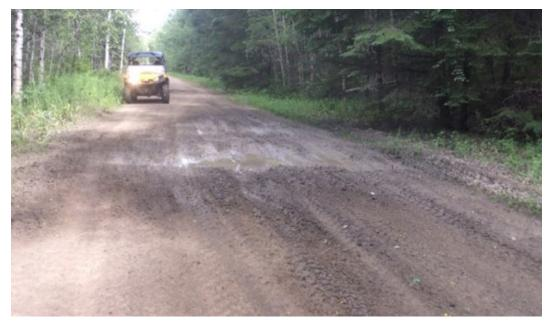
An area west of Lindbergh where the trail prism/crowned trail tread with adjacent ditches has not been maintained. Here the trail is cupped and the ditches are filled in and too far away from the ride surface.
