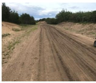
8m wide section of loose sand with washboard near Bellis
