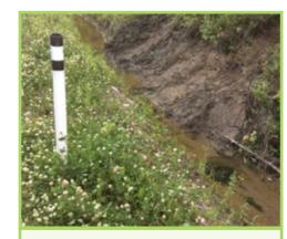
Narrow ditch is slumping and restrict water flow and volume
