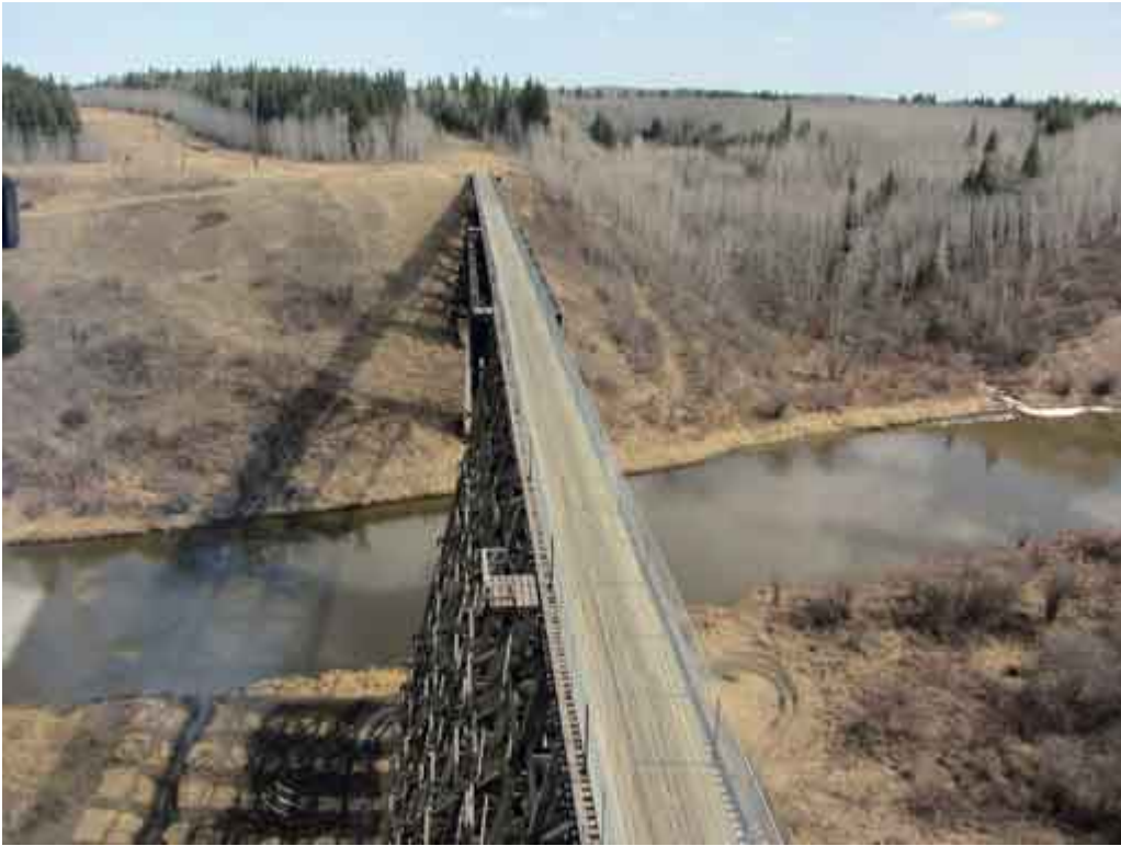
Trestle Before the Fire
