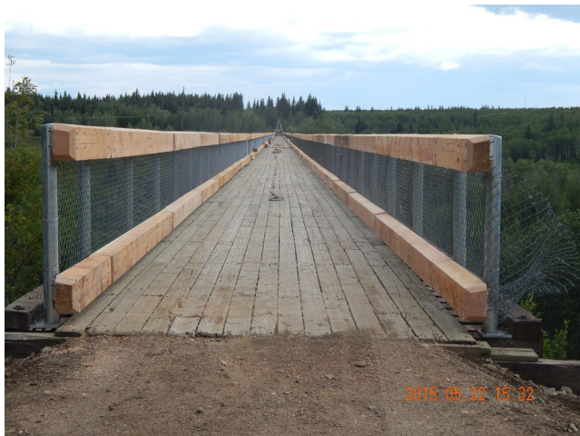
May June Repair of Railing
