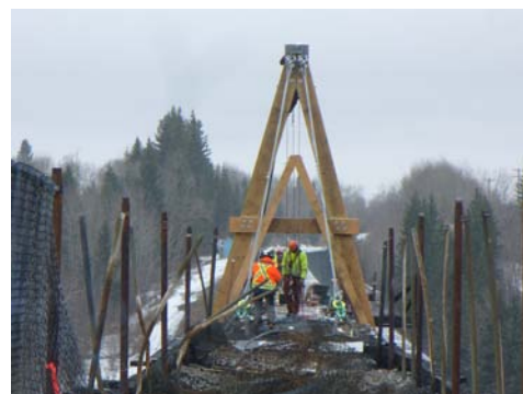
Burnt fencing, posts and upper deck.
