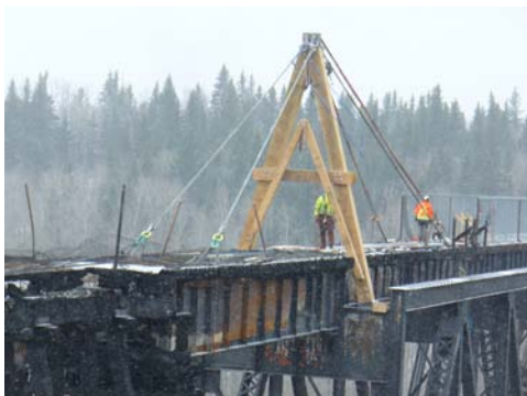
“A” frame construction to hold up steel girder.
