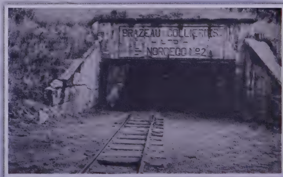
Brazeau Mine Portal #2
