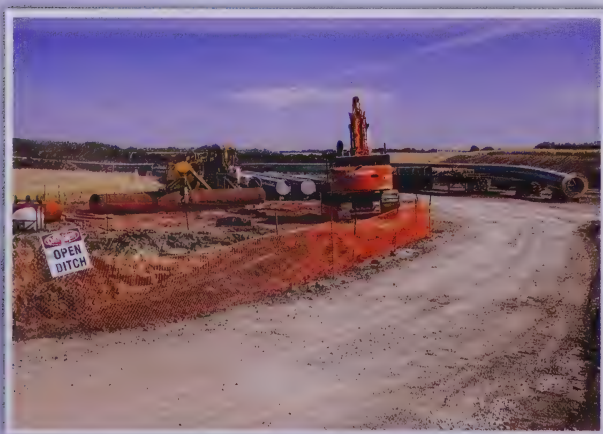
Pipeline construction north of Waskatenau. Photo-Carol Rusinek, Images Alberta
