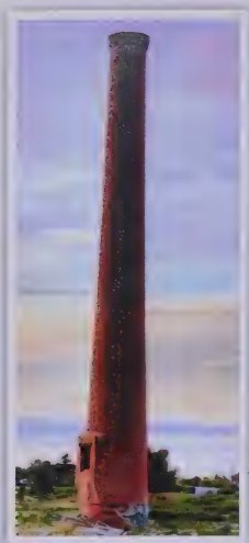
The largest brick chimney in western Canada, all that's left of the Canada Packers meat processing plant, 2013.
