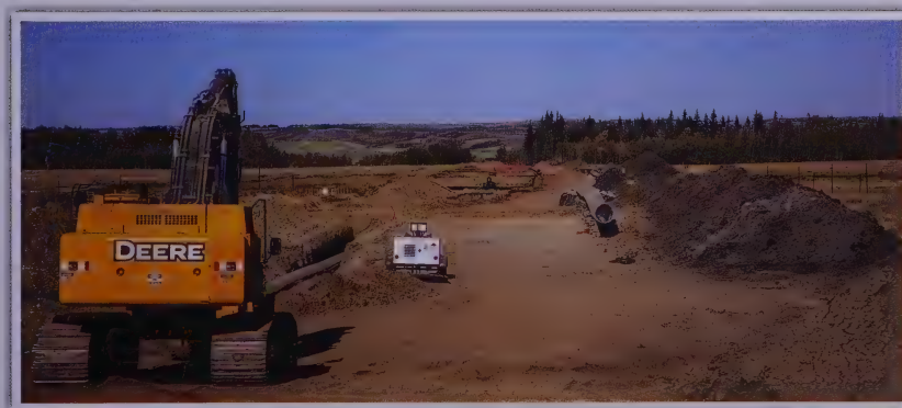
Pipeline construction in the Frog subwatershed in 2014. Photo-Bill Trout Images Alberta
